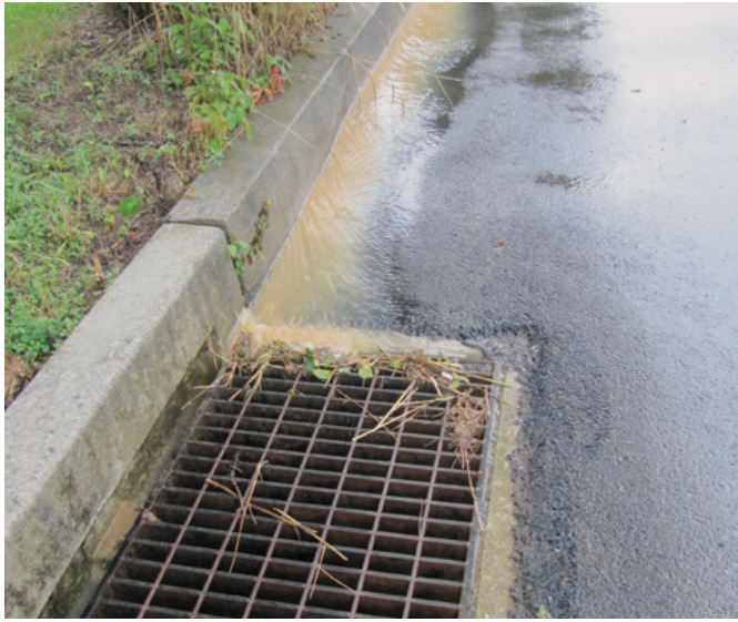
Figure 3b. Runoff that flows into storm sewer inlets eventually drains into local waterways. (Andy Yencha)
